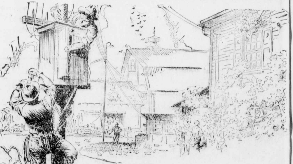
When rural service lines bring electricity to the farmer's door, many of his labor troubles are at an end. Motors, fans and small, will do the many chores of farm and farm house for a low cost per day.
