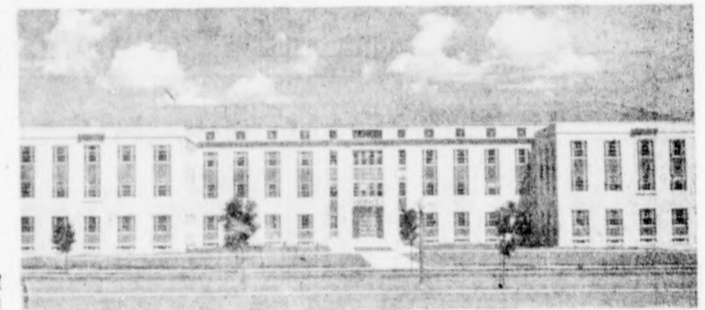
The new science building will celebrate its first official Homecoming with conducted tours through the interior of the building. Located on the East campus, the building was constructed at an estimated cost of $2,000,000. Final construction was completed last summer and classes moved into the building for the fall semester.
