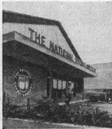
Our own network of stores—129 in the U.S., Canada and Venezuela—gives fast on-the-spot service to the oil fields.
