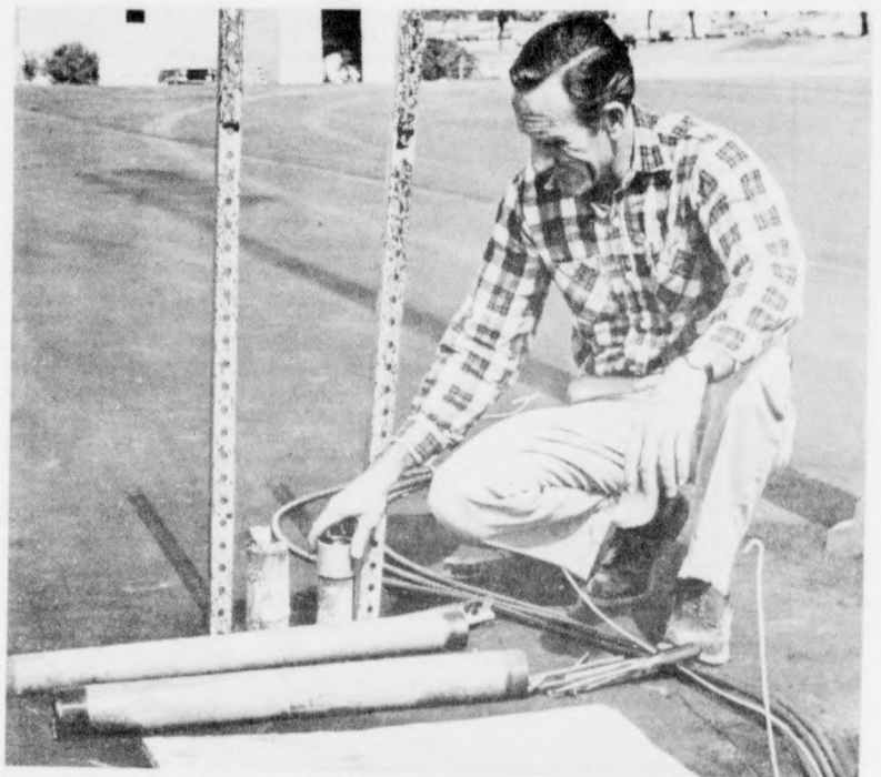
WORKMAN STARTS THE FINISHING TOUCHES FOR THE TENNIS COURTS
