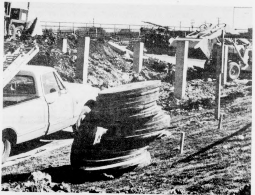
WORKERS DIG WORKING ON THE NEW ATHLETIC FIELD HOUSE
