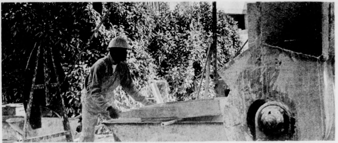
WORKERS MIX PLASTER Remodling continues on the Winton-Scott Science Building
