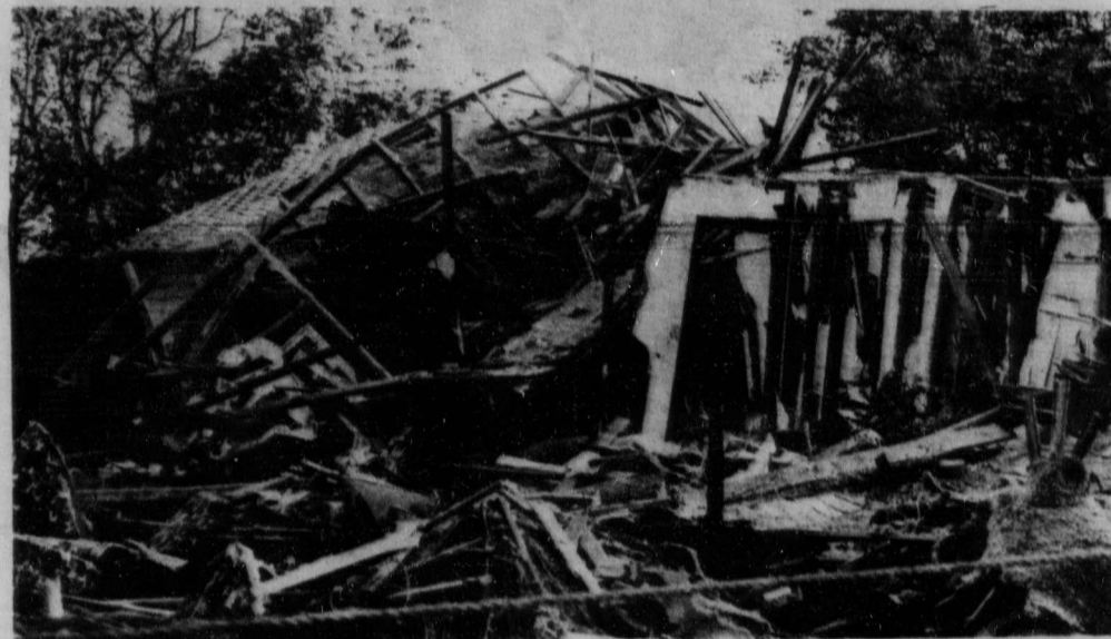
GAS LEAK?—This house explosion that killed a 62-year-old woman last week is being investigated by the
