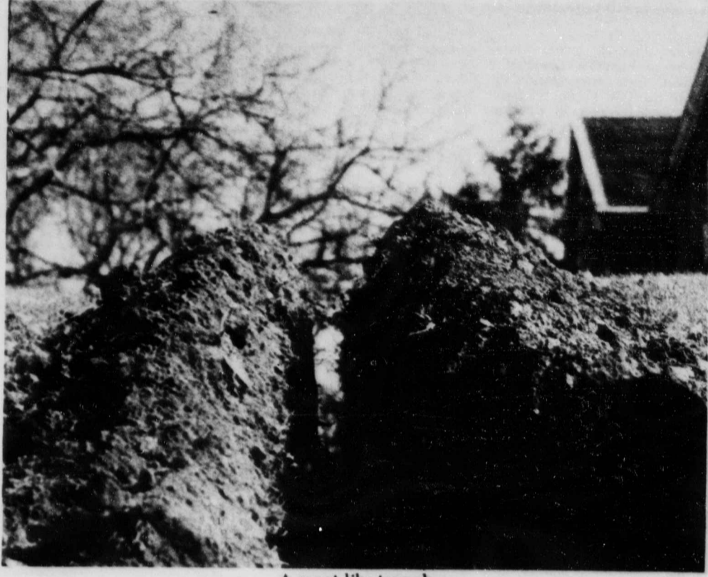
A moat-like trench
