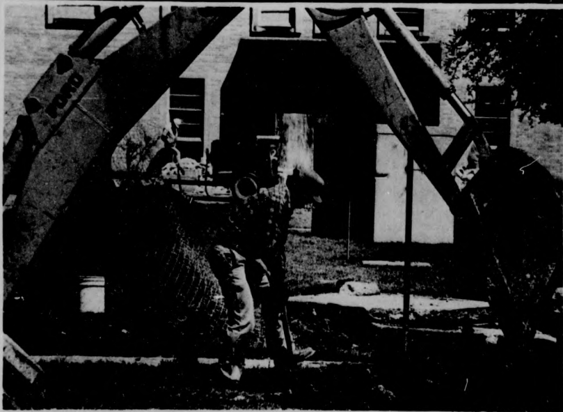
Minding his own business - R.H. Galloway of Century Mechanics digs a trench in front of Dan Rogers Hall for the sewer lines that will be needed for the new business building, Tandy Hall, Monday afternoon.
