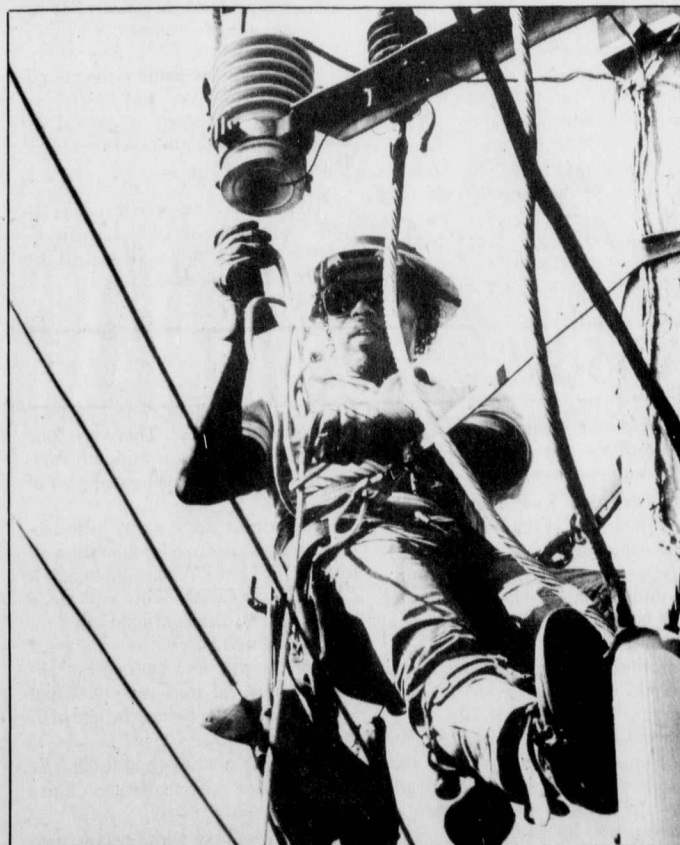
In charge - TU Electric restores power to Moudy Building after a squirrel caused a power outage.
