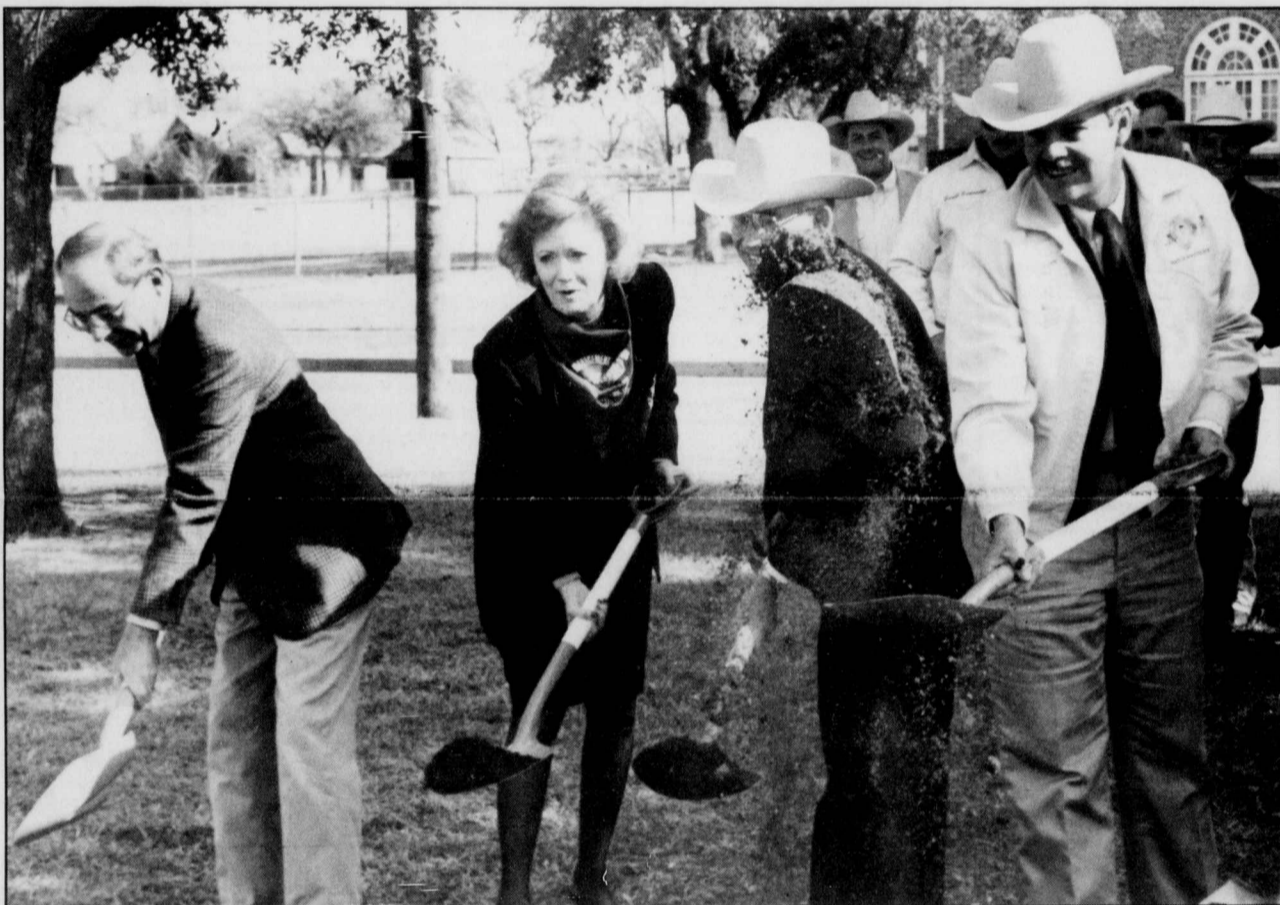
TCU Daily Skiff/ Aimee Herring With shovels in hand, Chancellor William Tucker, Fort Worth Mayor Kay Granger, Ranch Management Director John Merrill and philanthropist William Rockefeller lay the foundation for the future ranch management building. The new structure will double the existing space of the old ranch management building.
