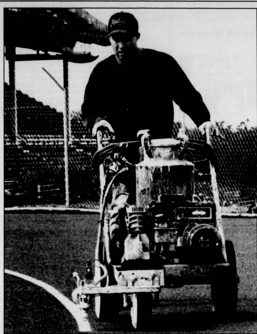
Chris Bullis paints lines on the track, which was just resurfaced. Bullis is with Vibra-Whirl, a Texas Panhandle company.
