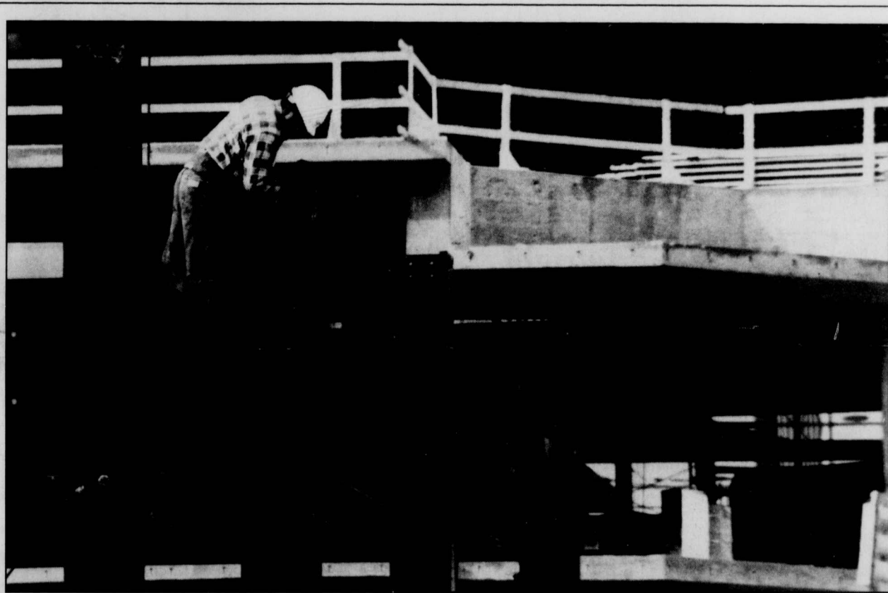
A construction worker checks the steel beams that will become the Nancy Lee and Perry R. Bass Fort Worth Performing Arts Center downtown.
