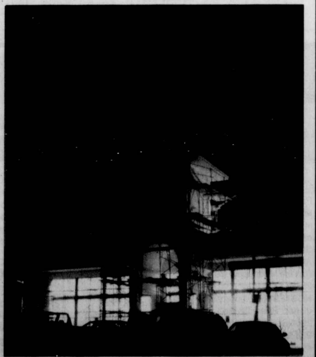
Construction workers toiled into the night Thursday to prepare the new bookstore for its opening Saturday. (Please see Perspectives pages 4 and 5.)
