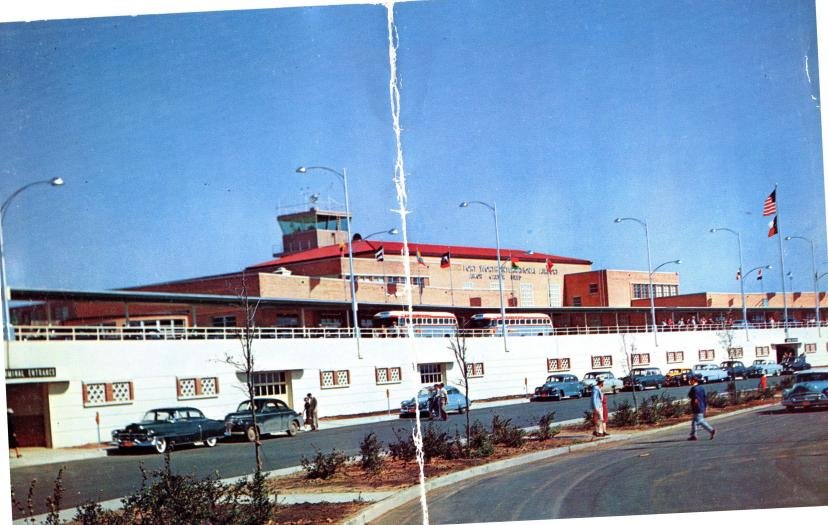
Seen in the foreground under loading and unloading ramp, is a storage garage for 200 automobiles available to air travelers. Traffic flows northward on the one-way ramp with facilities for enplaning passengers at the south end and deplaning passengers at the north. This great Air Terminal is located half way between Fort Worth and Dallas on Highway 183.
