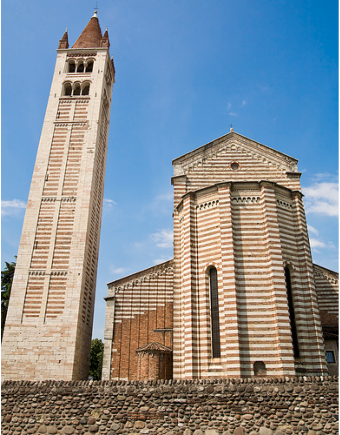
Figure 14 San Zeno Maggiore , Apse Exterior, Verona, Italy, completed 1398. Photograph by Andy Marshall (2007), http://www.flickr.com/photos/fotofacade/659951888/
