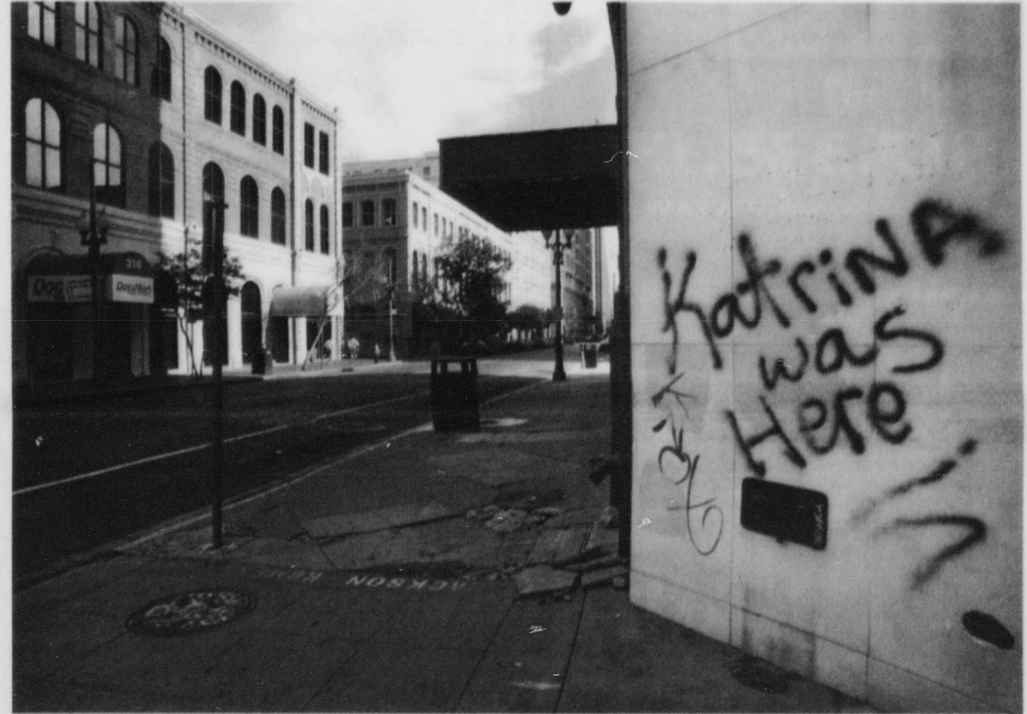
A message spray-painted on a building in downtown New Orleans in August 2005 was enough to explain what was responsible for the damage and the desolate streets. COURTESY OF MCT
