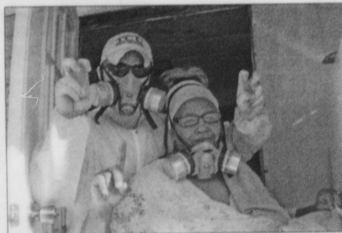
Noble helped rebuild the house of Salemah Broussard while he was in Lake Charles, La., for Spring Break. Noble was selected by ThinkMTV to help rebuild and repair houses damaged by Hurricane Katrina.
