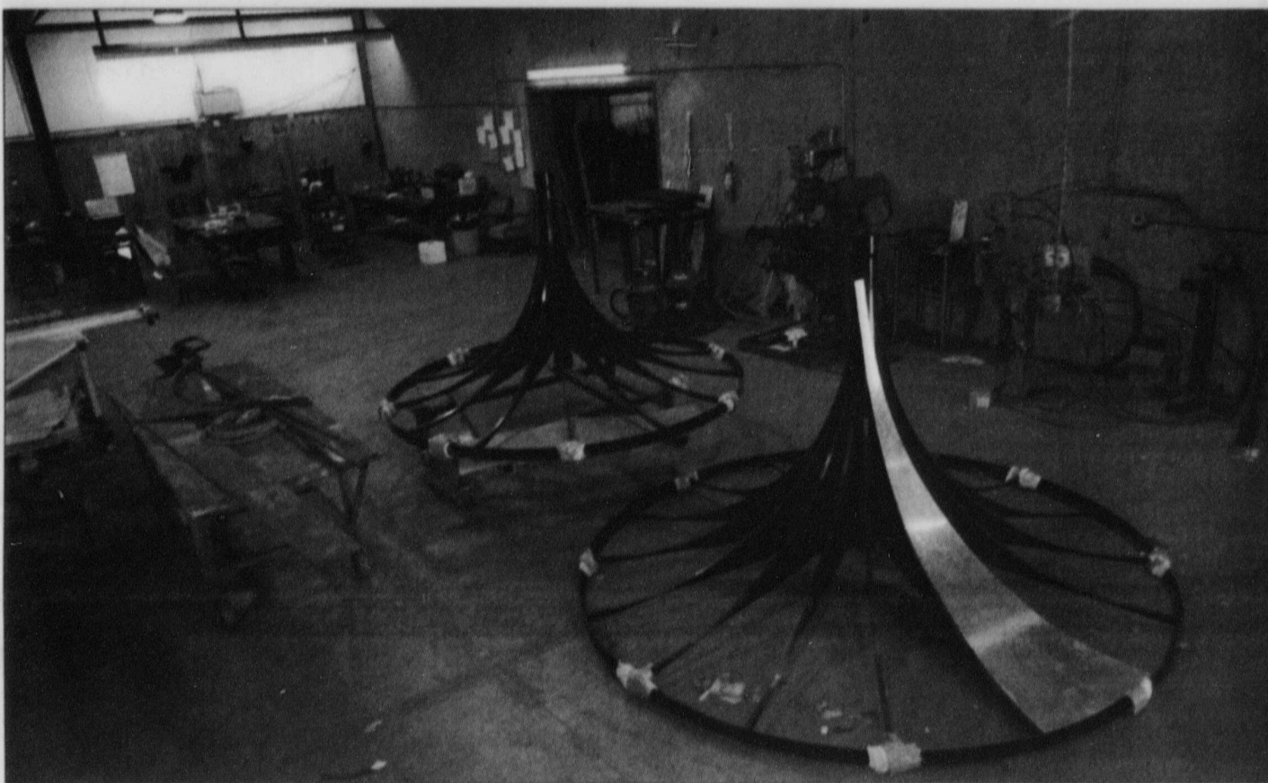
The new Frog Fountain lily pads sit partially completed at Kirby Sheet Metal on Tuesday. The pads need to have steel and a copper covering placed on top of the steel frame.
