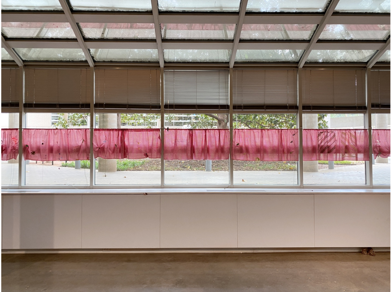
Figure 4: Installation view of North Tank
