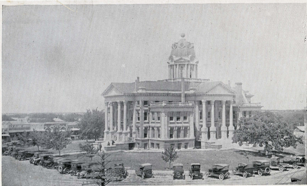
Court House, Montague County, Texas
