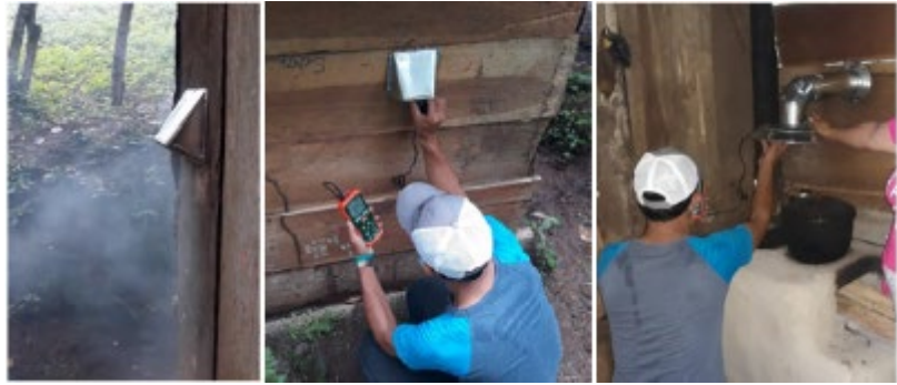
Figure 13: Installation and functional test of solar vents
