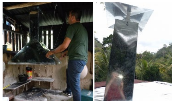
Figure 15: Redesigned hood and chimney ventilation unit
