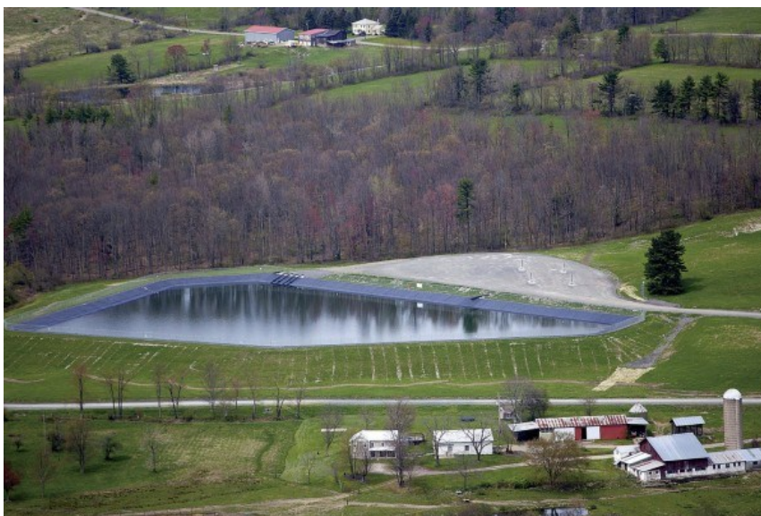
Figure 4: Wastewater Holding Pond for a Fracking Well in Rural Pennsylvania [2].
