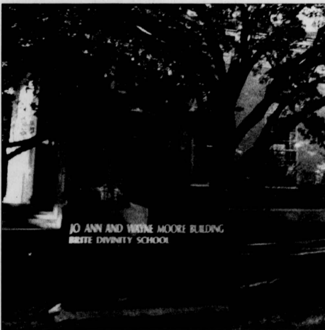
The Brite Divinity School building was renamed the Jo Ann and Wayne Moore Building during a ceremony Thursday. The Brite Board of Trustees will begin searching for a location for new housing facilities for Brite students soon.
