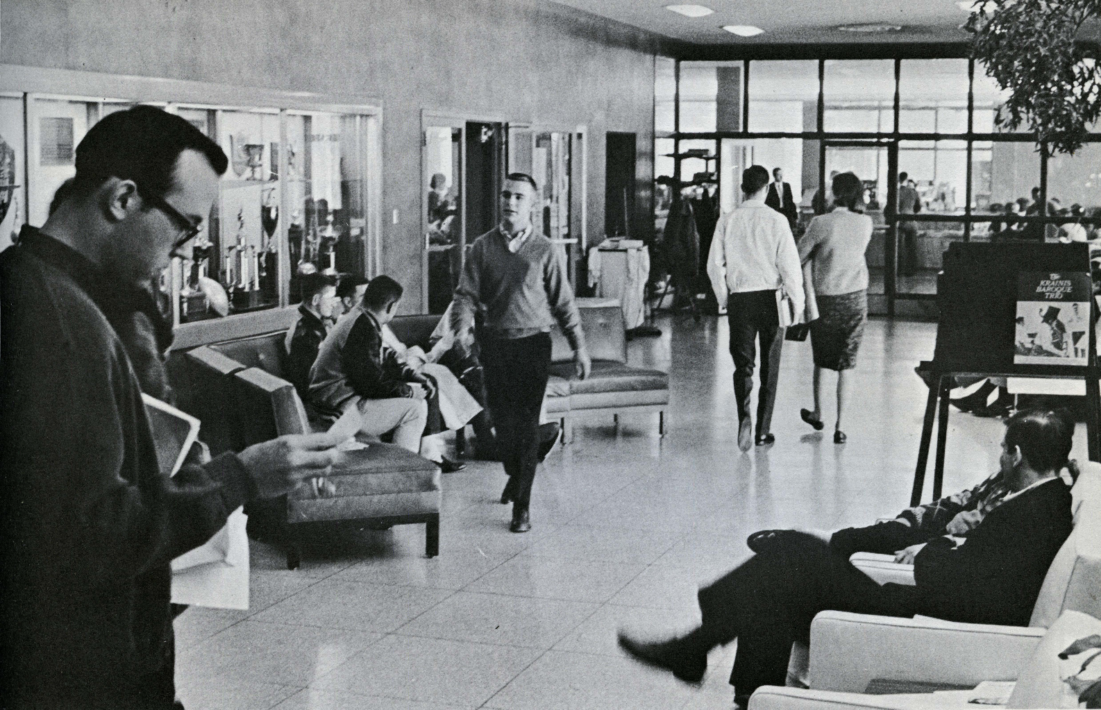
Busy lobby of TCU's Brown-Lupton Student Center.
