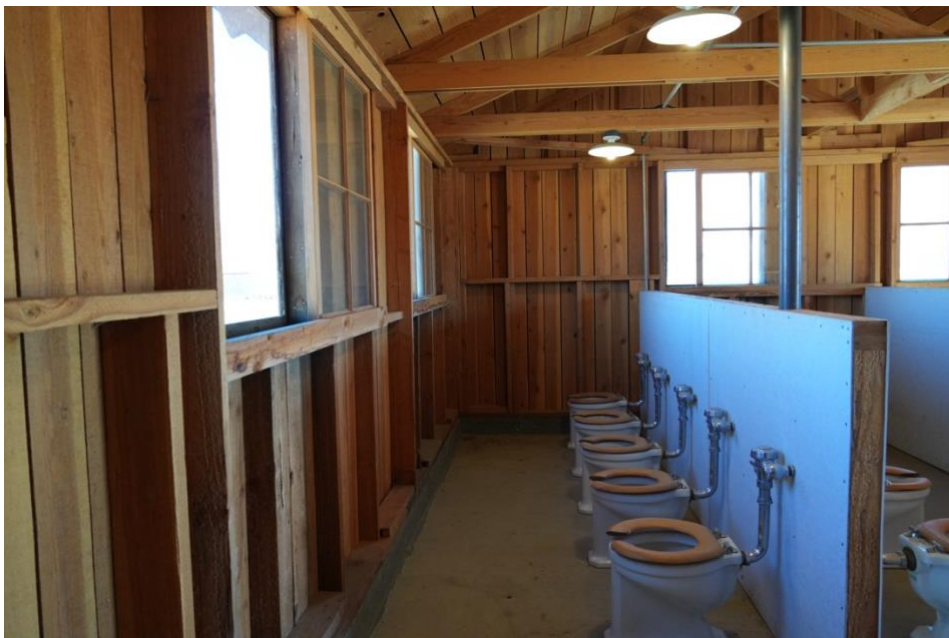
Interior of the women's latrine, note the lack of privacy barriers. Jan. 2025. Manzanar National Historic Site.
