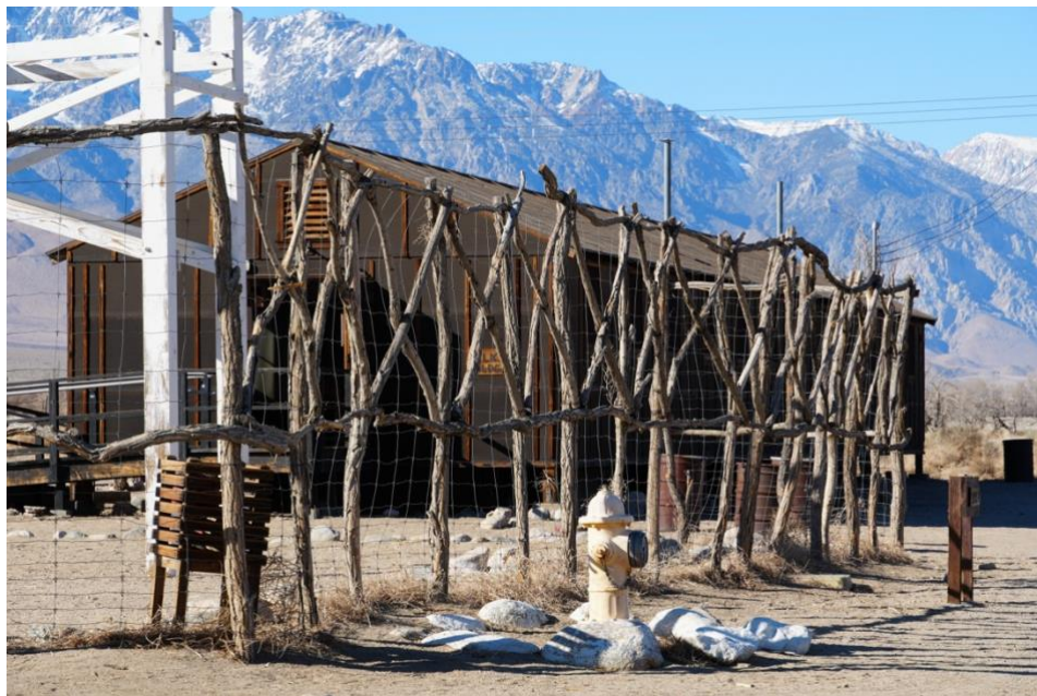
Reconstructed barbed wire fence which surrounded the camp. Jan. 2025. Manzanar National Historic Site.
