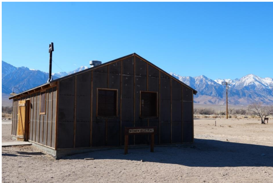
Exterior of the women's latrine. Jan. 2025. Manzanar National Historic Site.
