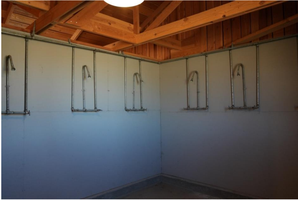
Interior of the women's latrine. Jan. 2025. Manzanar National Historic Site.
