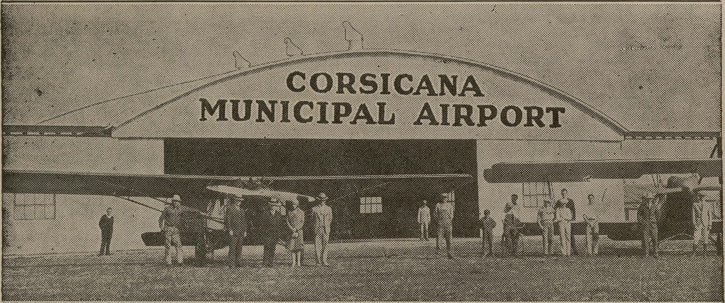
A view of the new $20,000 Municipal Airport at Corsicana, Texas, showing two of the planes operated at the port. The opening of the port was held April 27 and 28 with thousands attending.
