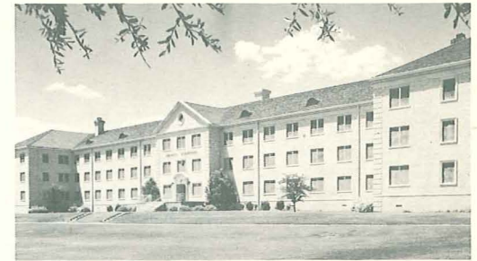
Exterior of Colby Hall Dormitory, where one of the receptions will be held on Thursday evening.
