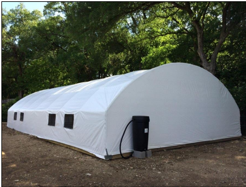
Figure 3. Exterior view of flight facility with custom-made screen windows.
