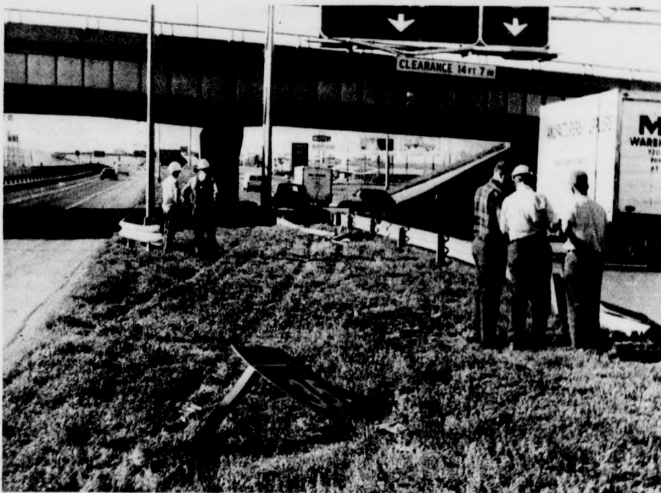
CRASH ROUTE—This photo shows the path taken by football coach Billy Tohill's auto when it left the roadway Wednesday morning and plowed through a variety of roadside barriers.
