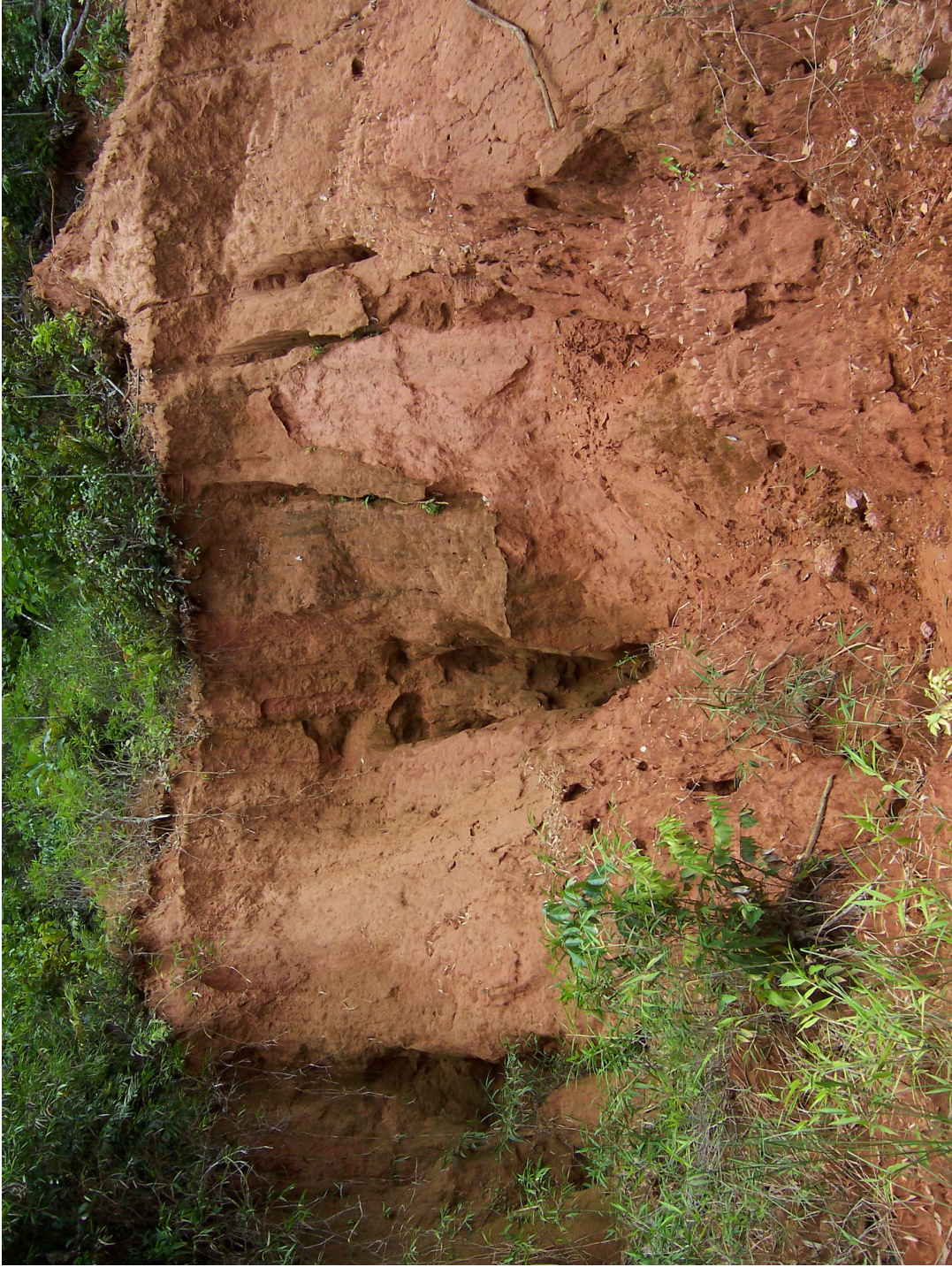
Fig. 2.6.5: Silty soils showing water erosion in exposed areas.
