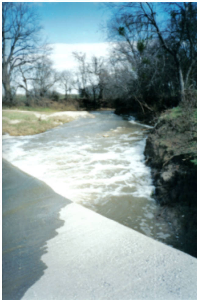
Spillway North of Sampling Site #1 – High Flow
