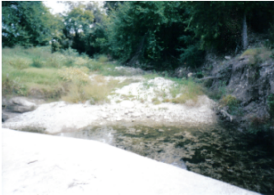
Spillway North of Sampling Site #1 – Low Flow
