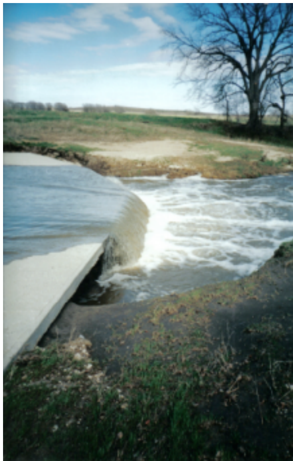
Spillway North of Sampling Site #1 – High Flow
