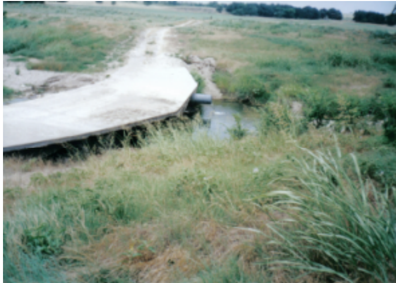
Spillway North of Sampling Site #1 – Low Flow
