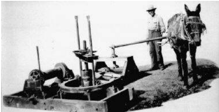
Figure 3 This photograph depicts the original water well being dug in which petroleum was discovered. Navarro County Historical Society.
