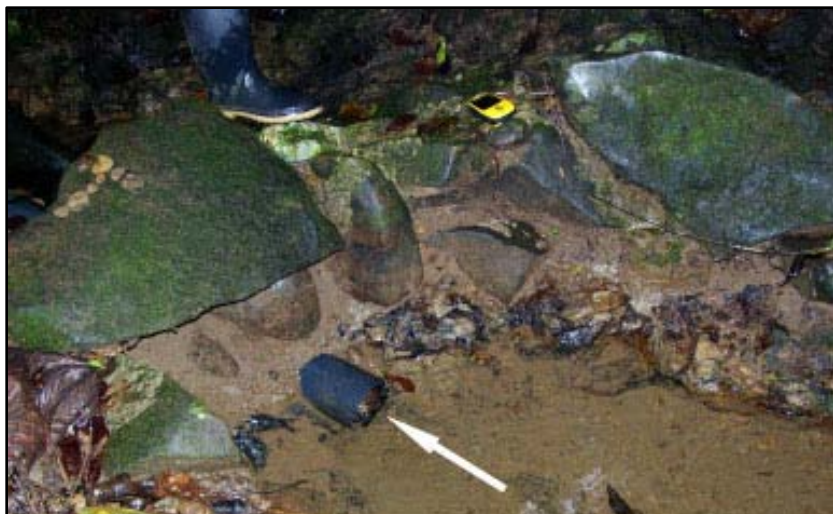
Figure 4: Water source for the houses and cabins. A small dam of rocks was constructed to pool the water, allowing a 3 ½" pipe to capture the water and send it to a holding tank. A similar structure is used at the water source for the research station, as well.
