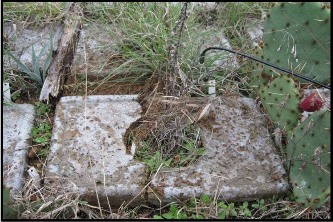
Figure 4: SM200 in the crack between the tiles.
