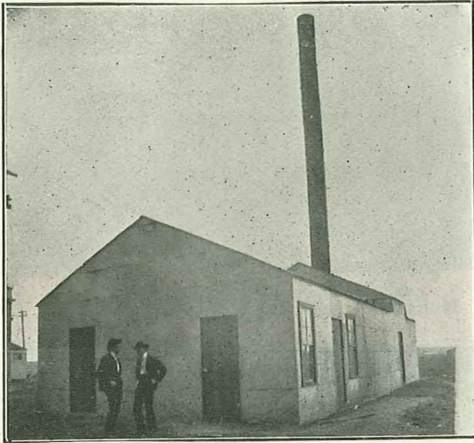
THE CENTRAL HEATING AND LIGHTING PLANT.
